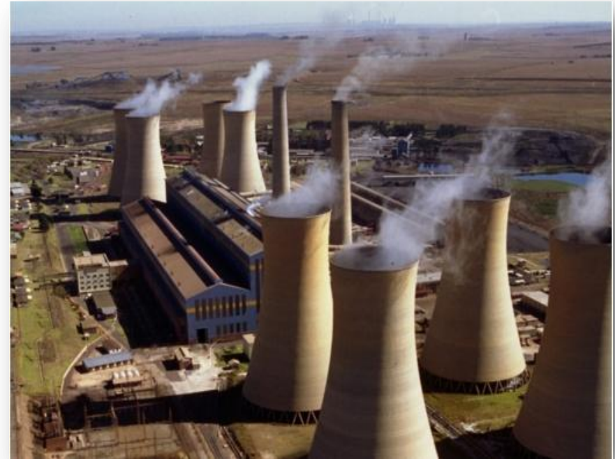
Komati Power Station
